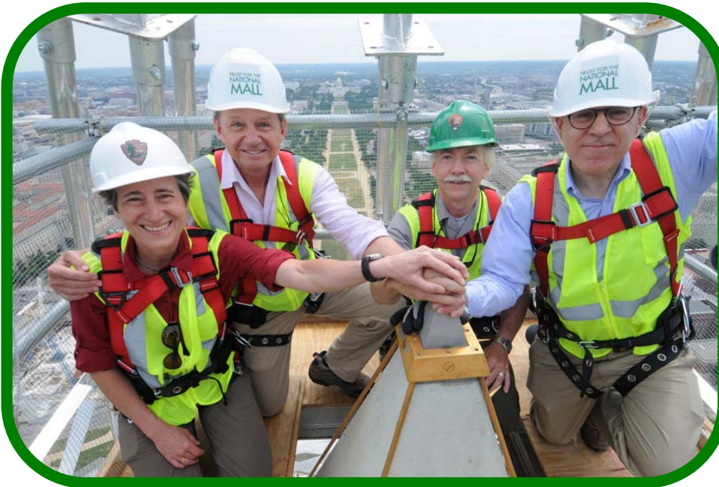
Interior Secretary Sally Jewell, along with John "Chip" Akridge, National Park Service Director Jon Jarvis and David Rubenstein touch the top of the Washington Monument. The Washington Monument is currently covered in scaffolding for repairs from an August 2011 earthquake. Photo: Tami A. Heilemann
